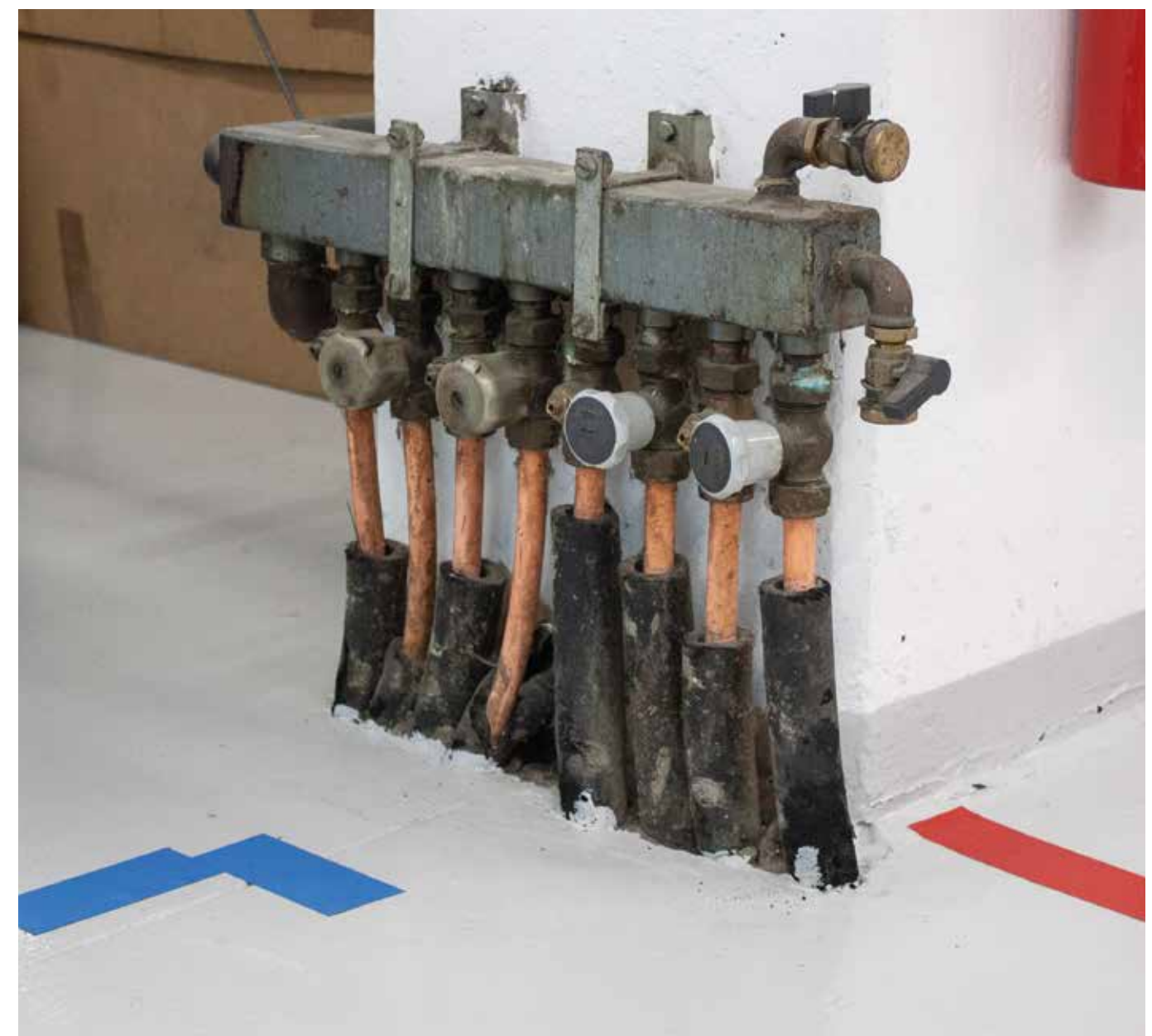
Floor heating in offices and production hall.
