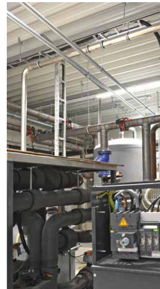
Air-source heat pump with adjacent „control center“
