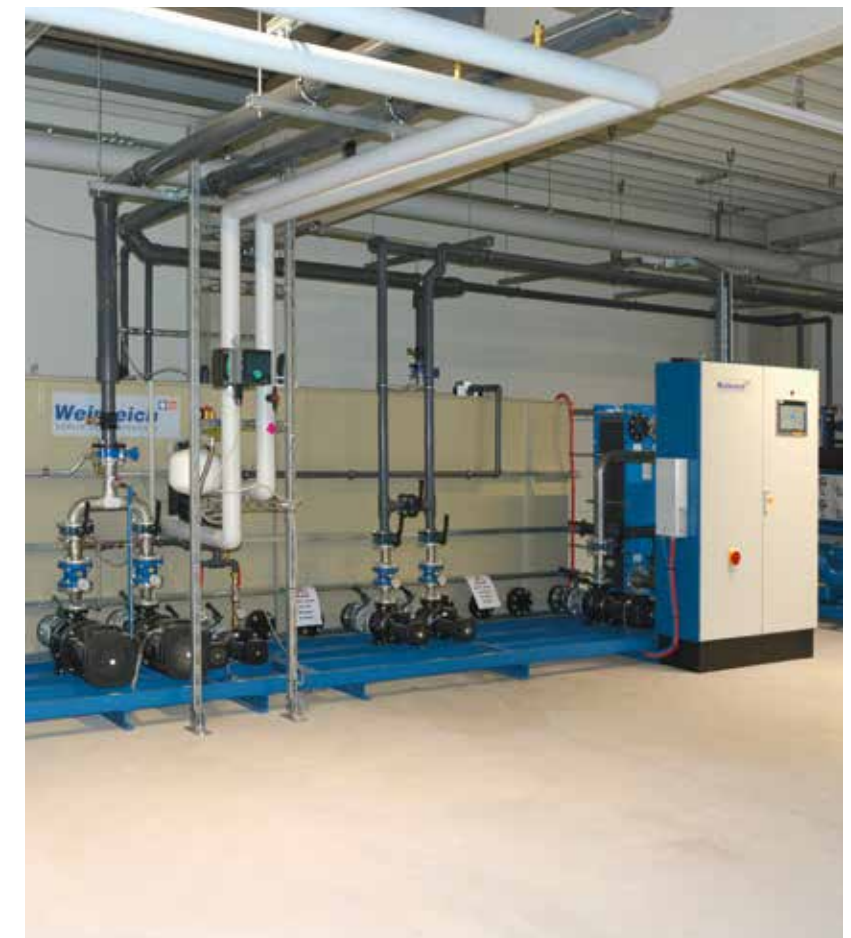
Cooling system for process cooling with heat recycling
