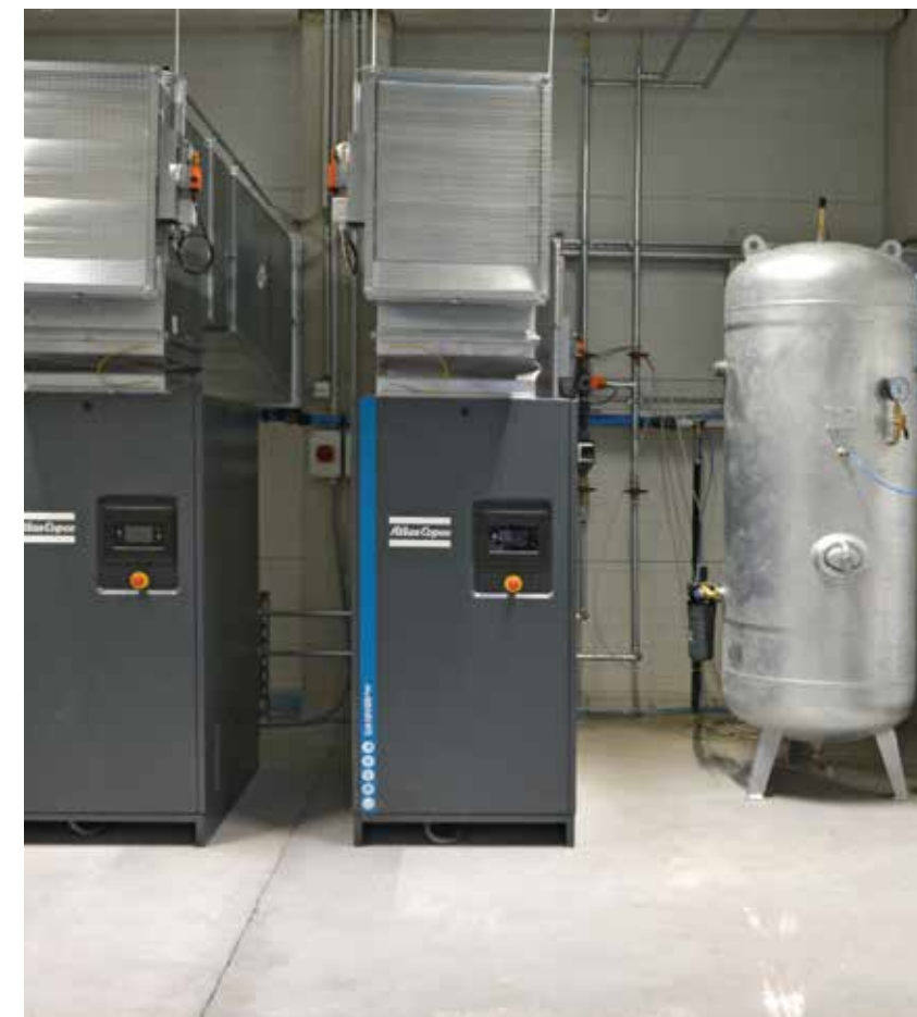
Compressed air generator with heat recycling
