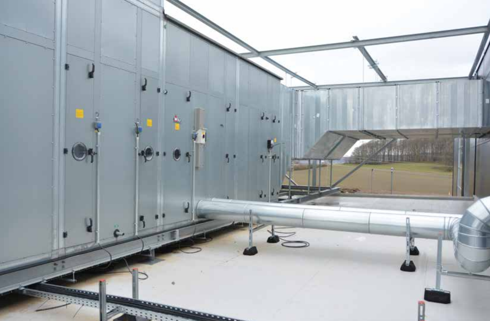
Outdoor ventilation system - 50,000 m 3 /hour with low vibration.
