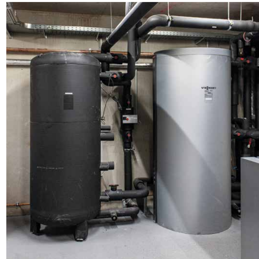
Stratified tank for Heating water
